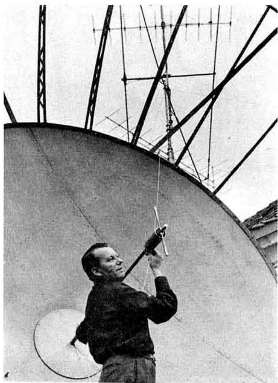
HB9RF adjusting the 432 Mc/s dipole on his dish aerial. (Photo via G2AIW)
